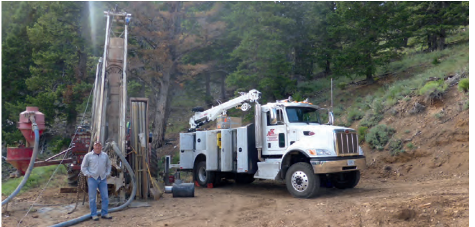
Drilling at Empire
